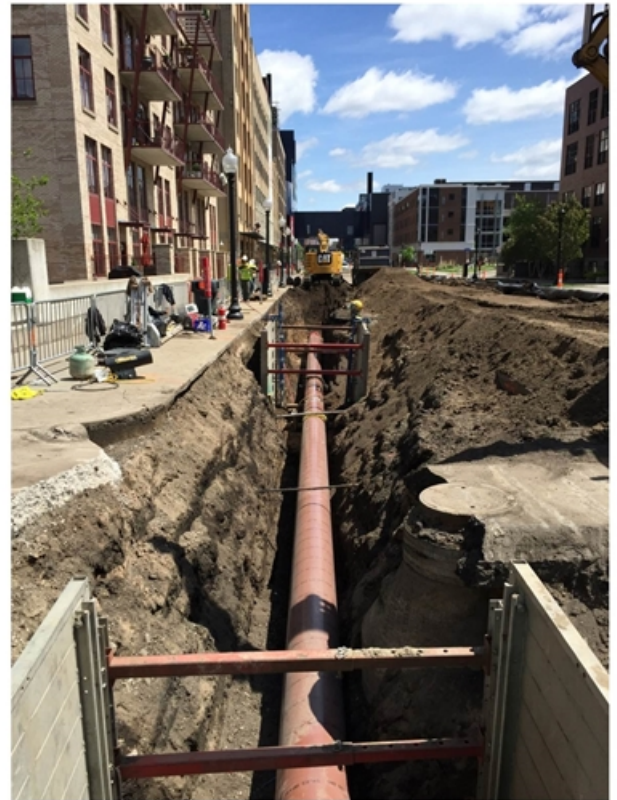
2015 Minnesota Beltline Replacement Project in downtown Minneapolis
