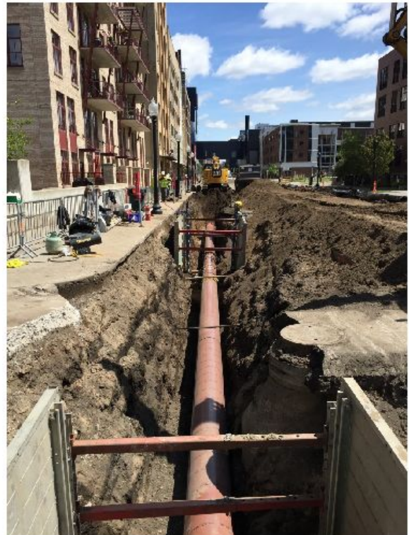
2015 Minnesota Beltline Replacement Project in downtown Minneapolis
