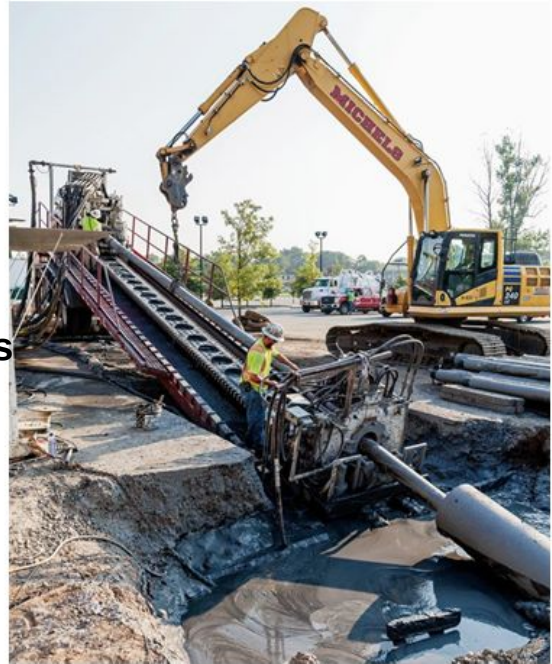
Using horizontal directional drilling to construct and install a new pipeline under the bed of the Arkansas River
