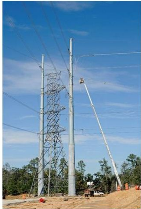
Construction of high voltage transmission infrastructure
