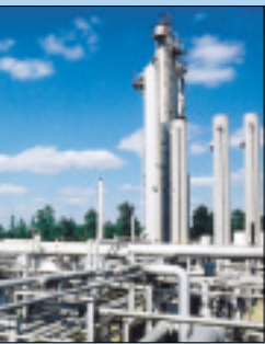
THE PERLA, ARK., STATION IS A VITAL PART OF PIPELINE OPERATIONS.
